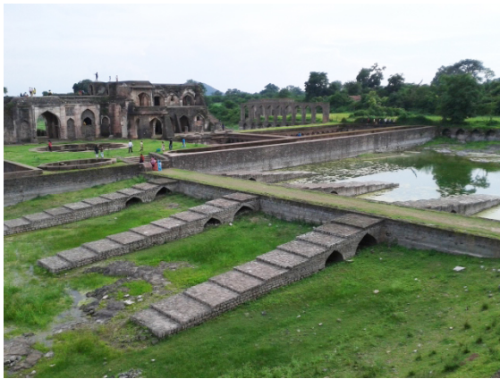
Fig. 6. Rain harvesting and accessing systems, Mandu Fort, M.P. Picture Credit: Poonam Verma Mascarenhas.
